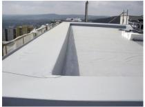
The attic during the renovation - installation of additional thermal insulation over the attic to reduce the thermal bridge (left) and a view of the new waterproofing/covering layer made of mPVC sheets (right). Precise design and construction of structural details are crucial for proper function of any energy efficient building. [1]
