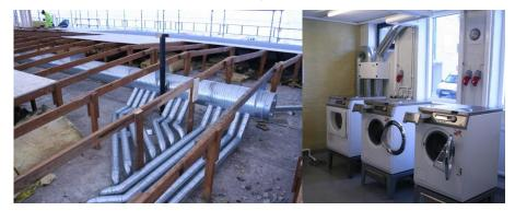
Installation of ventilation ducts in the new attic and new washing machines in the common laundry room.
