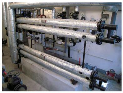
Original heat exchangers in the boiler room (before renovation). [2]
