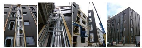
Different steps of the building renovation process: installation of the building services, assembling of the prefabricated façade modules, almost finished building envelope (f.l.t.r.)
