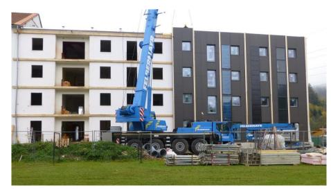
Assembling of the prefabricated façade modules on the west facade
