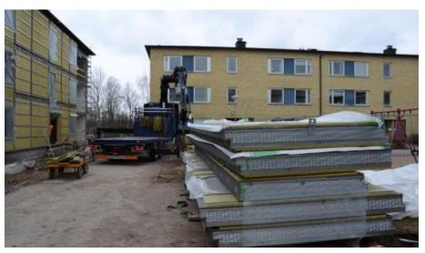
Prefabricated facade elements for the next phase of renovation.
