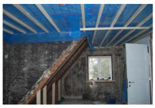
The new vapour barrier on the loft
