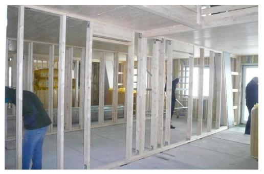
New internal walls and inserted deck at the first floor of block B.
