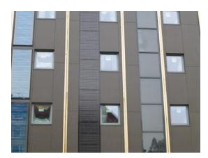
Prefabricated façade elements with integrated active energy production (photovoltaic and solar thermal panels)
